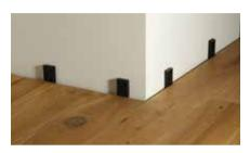
To allow for expansion gaps, spacers should be used at regular intervals when fitting and then removed before skirting boards, beading or trims are put in place.
