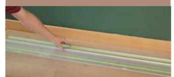
4. Using a blade that is the same width as the design strip, cut into the floor approximately Imm deeper than the design strip.
