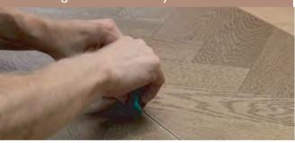
7. Apply a thin bead of PVA into the groove and insert the design strip.
