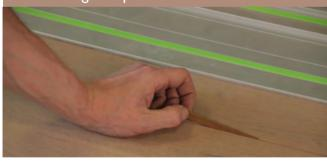
6. Run a piece of sandpaper over the top of the edges to remove any burrs.
